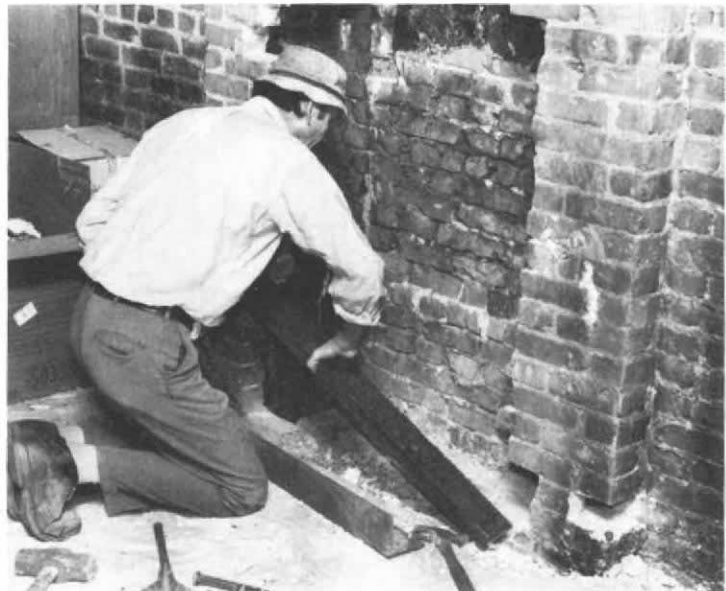
The first step in installing new flue liners is removing bricks from the second-floor fireplace to expose the chimney cavity. Hammer, railroad spike and pry bar are essential tools. A vinyl-covered canvas dropcloth over rubber carpet padding protects the floor. At right, Kitchel aligns two pieces of angle iron, which will be cemented in place across the face of the cavity to reinforce the chimney before the new liner is installed.
