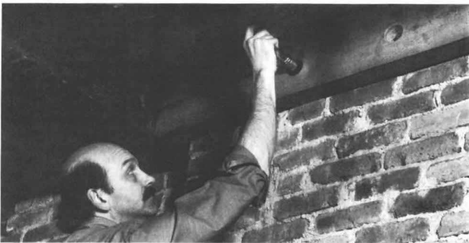
A plywood sheet, top, temporarily replaces the third-floor hearthstone. The face course below has been relaid using the original bricks and repointed to match the style of the original chimney. Above, bolts sunk in the reconstructed face course just below the third floor secure a new chimney girt, to the wall. This will support a new section of floor that replaces the third-floor hearthstone.
